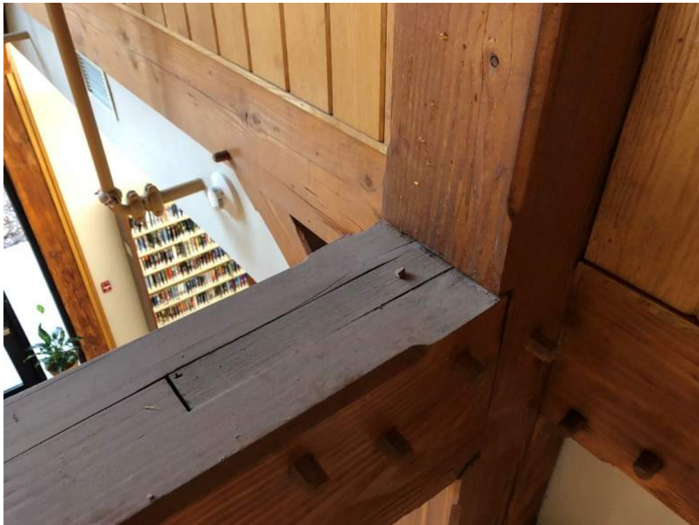
Photograph 14: Typical mortise and tenon timber frame joinery.
