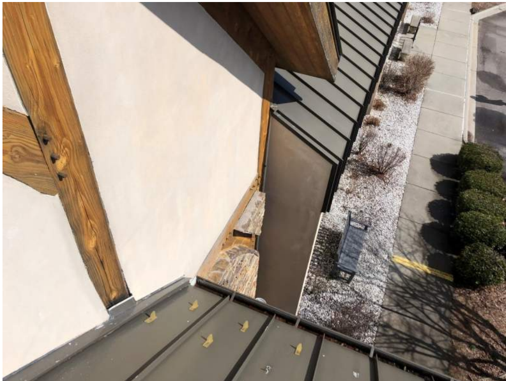
Photograph 7: Exterior cladding has been pulled away from the building by the connector roof.
