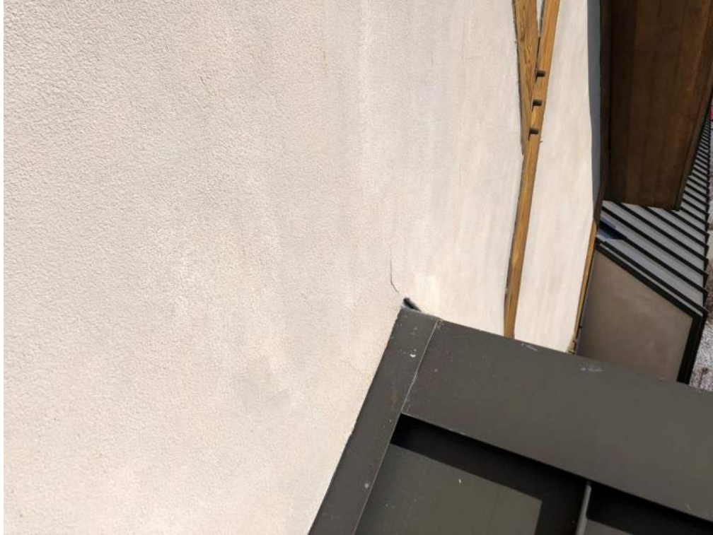
Photograph 7: Exterior cladding has been pulled away from the building by the connector roof.
