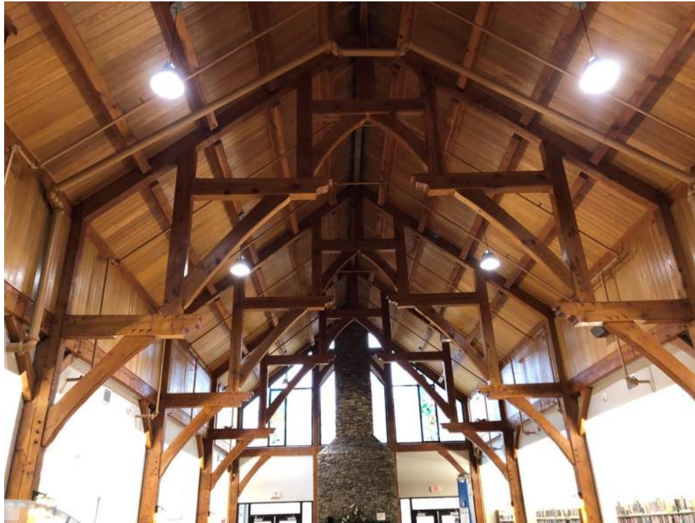
Photograph 11: Timber 'hammer' frames in the Lobby area.
