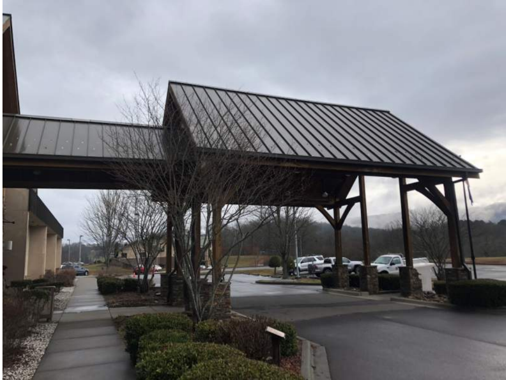
Photograph 1: Existing Porte Cochere.
